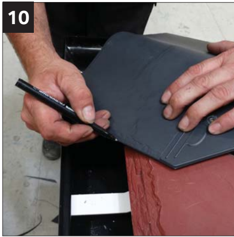
10 Mark the position of the edge of the tile starter on the hip tile at the outer edges and in the middle/
