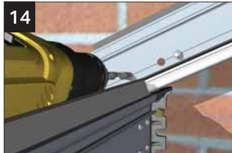
Drill an 11mm hole through the aluminium starter and its factory inserted reinforcement. Then use a 10mm masonry drill bit for the host masonry.
